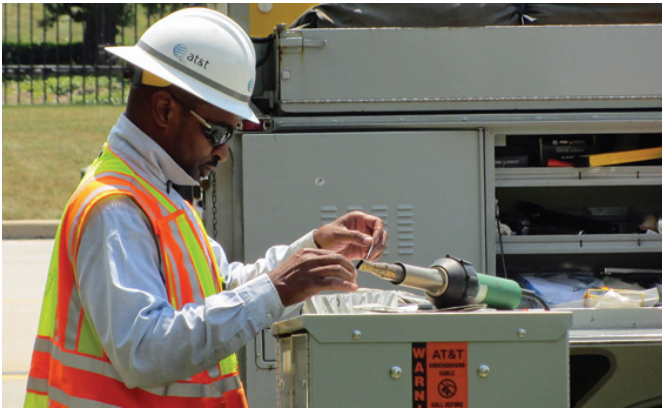
Steve McCullum - Romeoville DEG tech working on a crossbox in Alsip.
